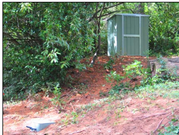
Figure 2.4: Katoomba, NSW Test Site Installation
